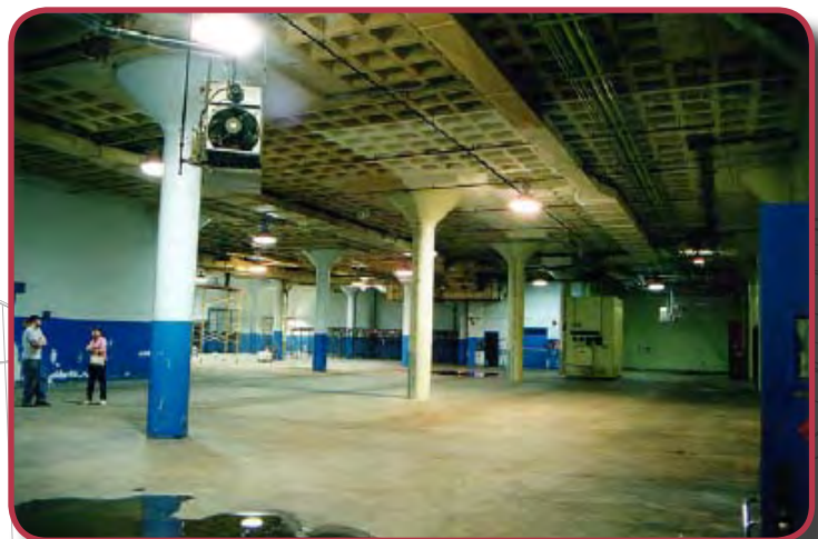
Fig. 1.3 we had to measure out this 40,000 square-foot facility now known as East Coast Terminal
